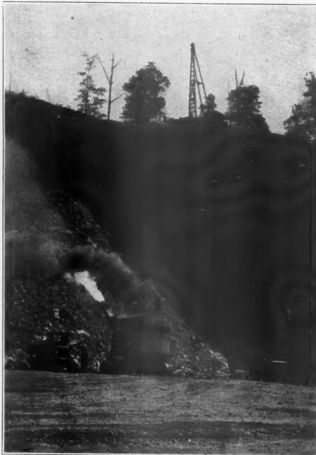
Breast of Quarry Showing Steam Shovels at Work and Drill at Top of Deposit
